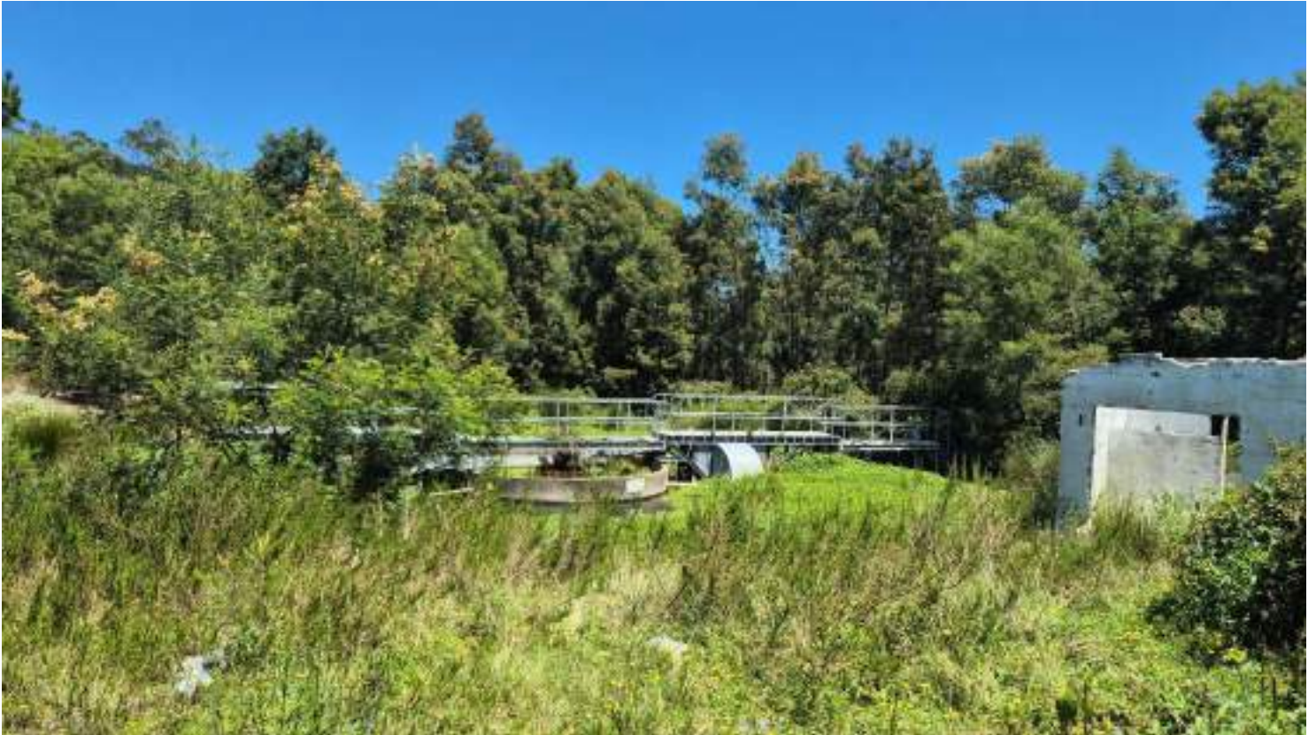
Figure 5.10 Existing WWTW facility in the southwestern part of the development area.
