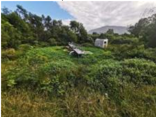
Figure 20: Current WWTW, overgrown with weeds.
