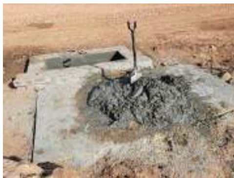
Figure 17. Example of mixing cement (dagha) on a wooden board to prevent wash off to watercourses during rainfall.
