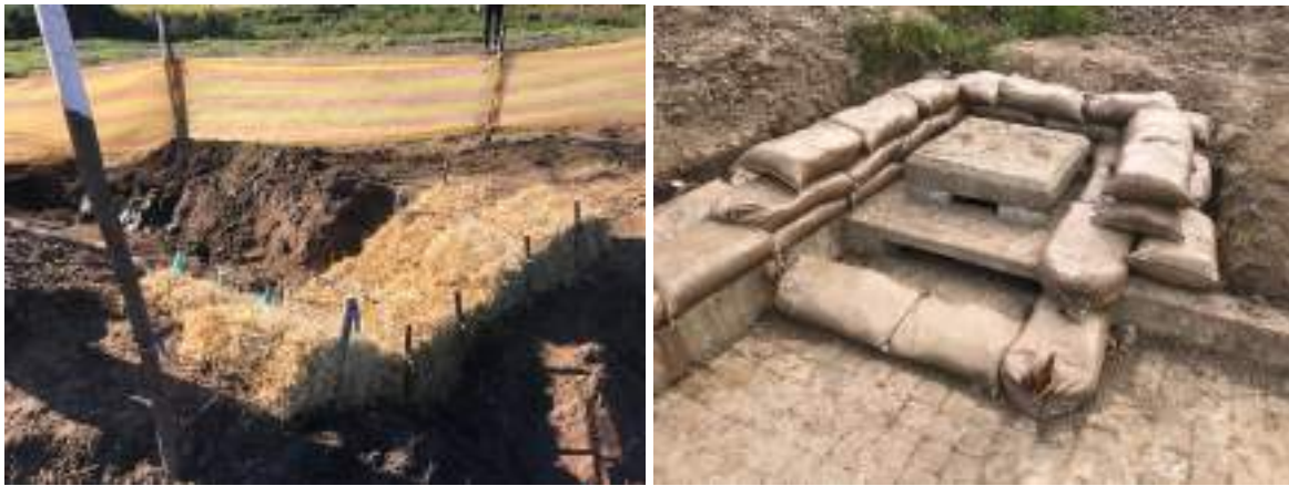
Figure 19. Examples of a haybale check dam in a concentrated flow path (left) and sandbags surrounding a stormwater drain which leads to a wetland. This prevents silt laden water from entering the wetland where it would be difficult to remove.
