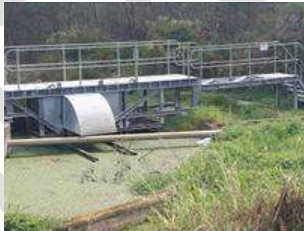
Figure E Pedestrian Bridge
