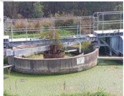
Figure F Pedestrian Bridge
