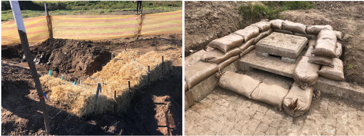
Figure 19. Examples of a haybale check dam in a concentrated flow path (left) and sandbags surrounding a stormwater drain which leads to a wetland. This prevents silt laden water from entering the wetland where it would be difficult to remove.
