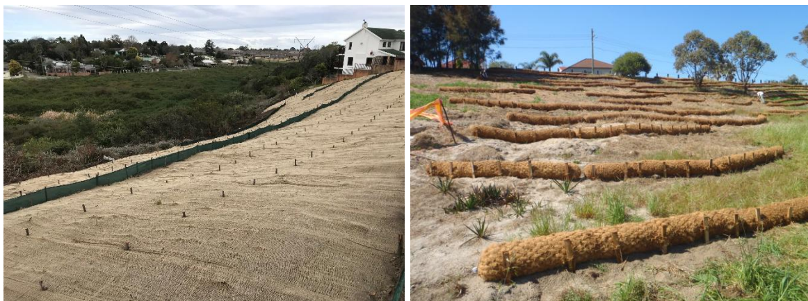
Figure 18. Examples of silt fences with soil saver matting (left) and coir logs (right) used to trap sediment mobilised from steep slopes during the construction phase.
