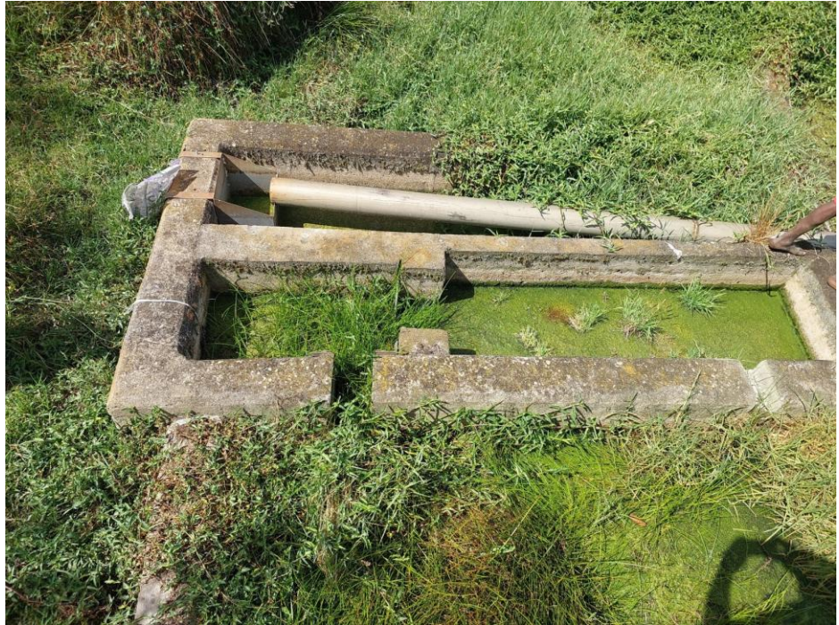
Figure C Overgrown Sedimentation Tank
