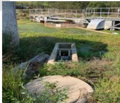
Figure H Overgrown Sedimentation Tank
