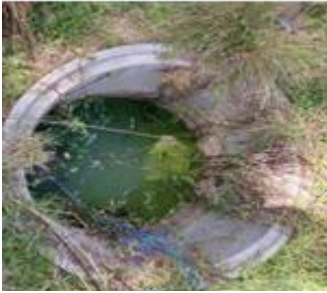
Figure A Overgrown Manhole
