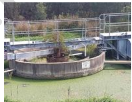
Figure F Pedestrian Bridge
