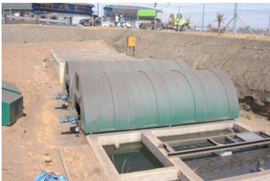
Figure 3-4 Typical layout for RBC
