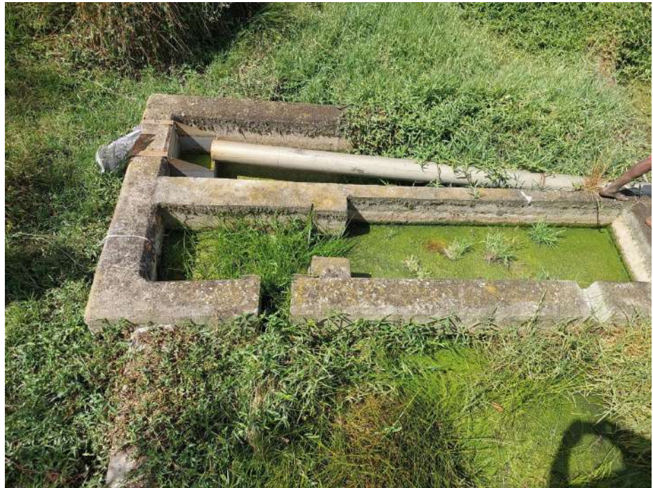
Figure C Overgrown Sedimentation Tank
