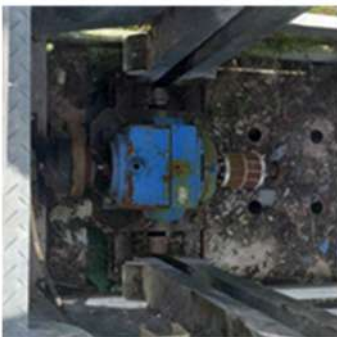
Figure D Corroded Motor
