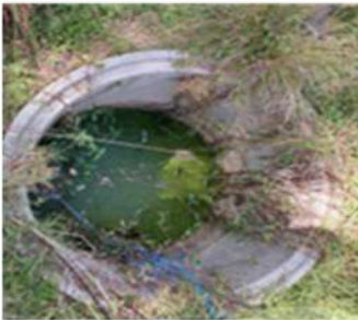
Figure A Overgrown Manhole
