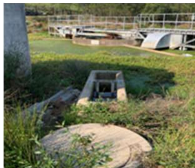
Figure H Overgrown Sedimentation Tank
